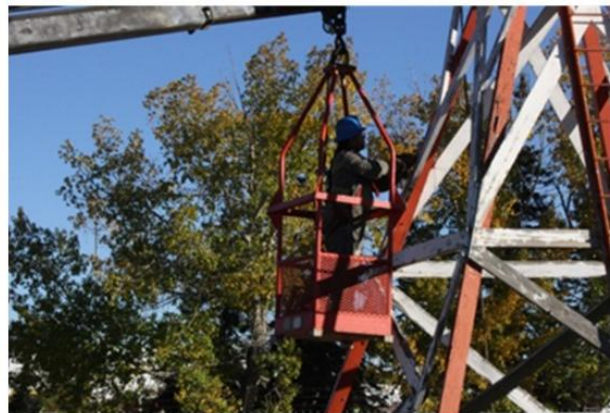
Cutting the cupola off the tower
