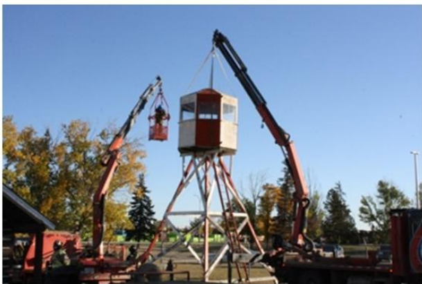
Hooking up the straps from the boom
